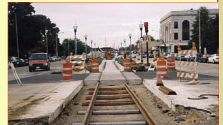
By using steel ties where track runs through pavement, the cost of the in-street track was reduced.
