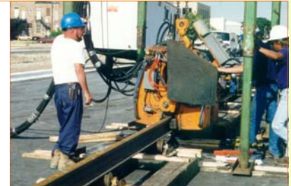
Electric flash-butt welding of rail to provide cost effective continuous welded rail (CWR)
