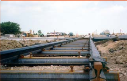
Embedded track construction with new continuous welded rail wrapped in the Ironhorse "Boot"®, fastened to steel ties.
